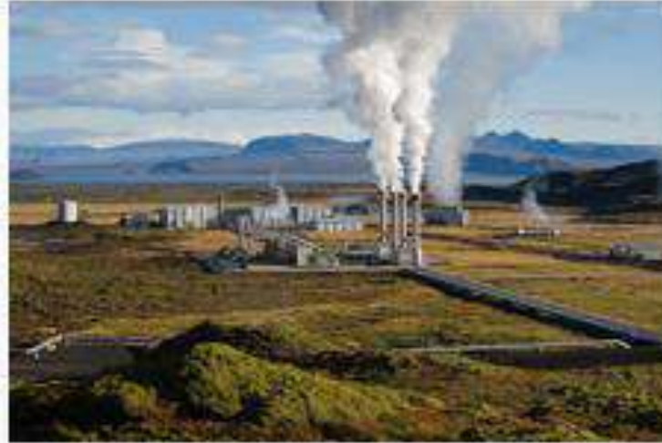
Nesjavellir Geothermal Power Station, Iceland
